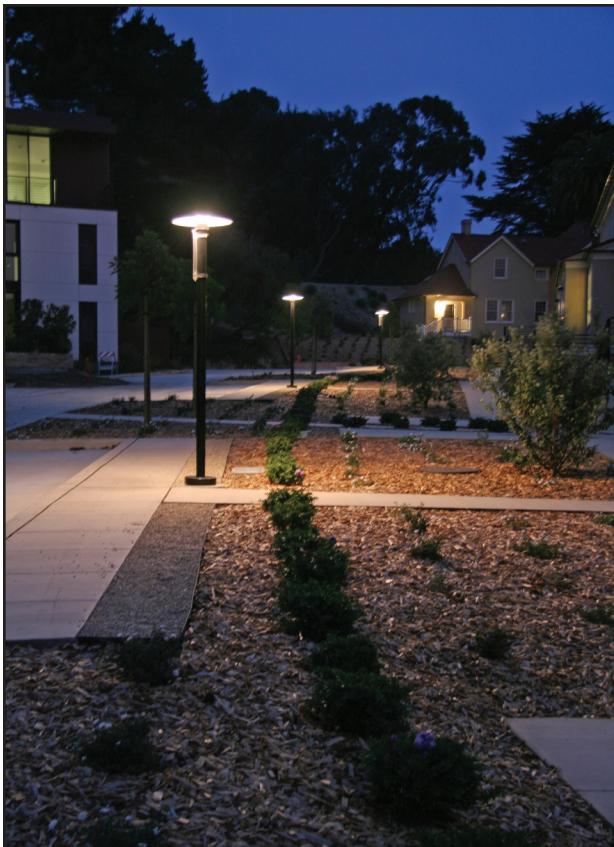
Note that the fixtures are 75 feet apart.
